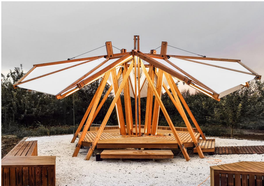
Figure 1. Roof fully open. By Feng Deng
